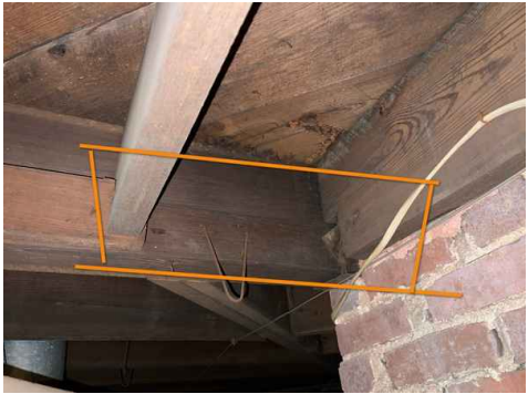
Missing Ledger Strip
